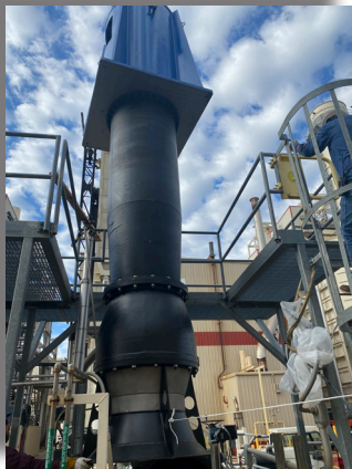
Power Generation Circ Water Pump
